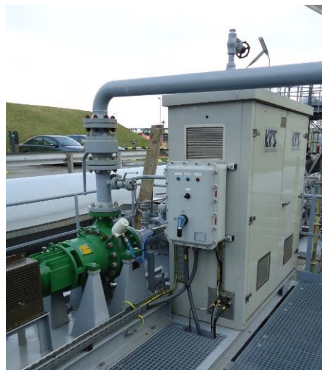
Figure 14: Field installation of e-Jetmixer
